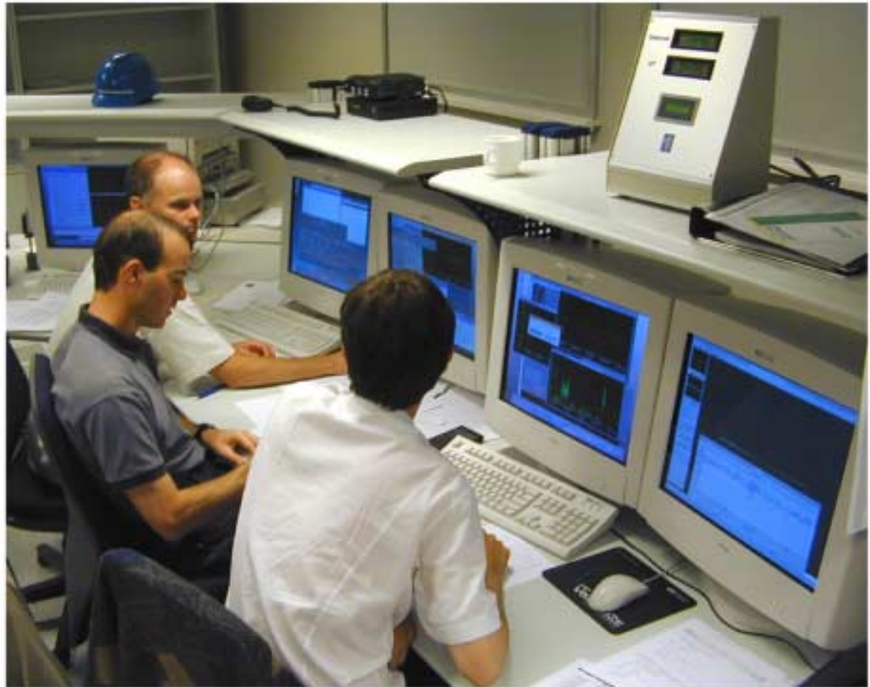
The VLTI Control Consoles
