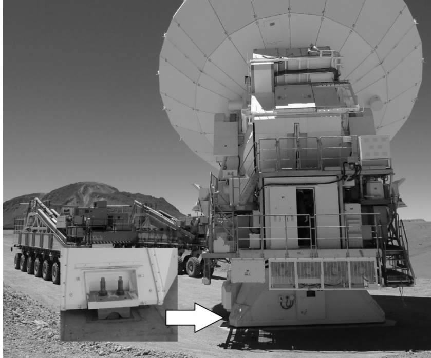
2 Antenna Installed on foundation with Interface detail
