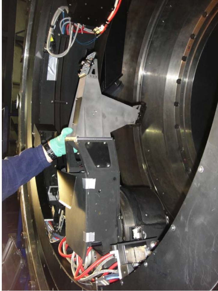
Figure 14. Photo taken while the installation of the new supporting arm on the sensor arm. Once removed the original sensor arm and checked space and interfaces it continued the installation.
