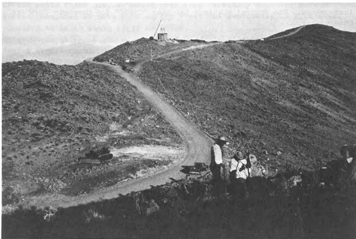
Fig. 2 Erection of building for 40-inch telescope.
