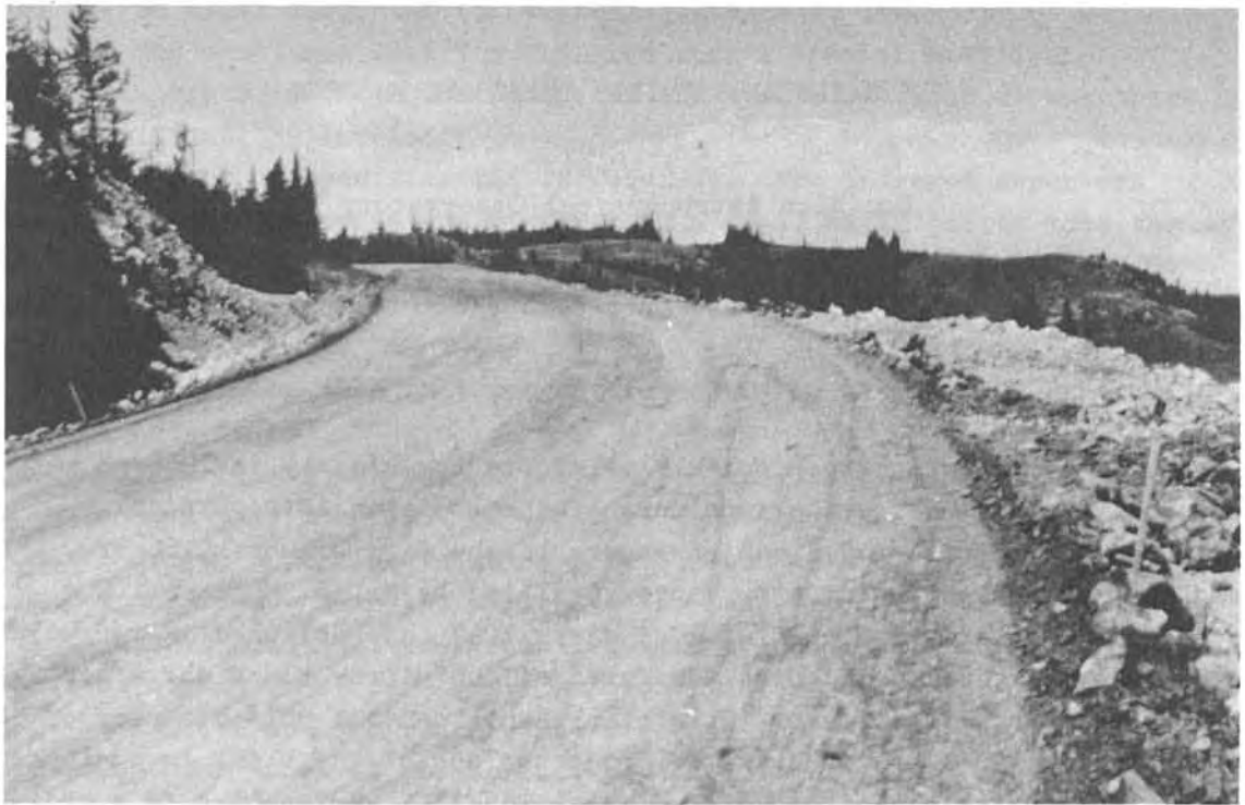
Fig. 1 Mount Kobau access road.
