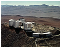
Figure 1.1 [JPG: 256k]. An aerial view of the Paranal summit in mid-April 1998 with the large observatory platform on which the many components of VLT were being installed. The four enclosures (telescope 'domes') are seen, three of which have been closed. The long, subterranean interferometric tunnel is in the middle. The concrete supports for the smaller, moveable telescopes of the VLT Interferometric Array are located all over the platform, together with the foundations for the tracks. The VLT control building, from where the observations with the four large telescopes will be made, is placed on a smaller and slightly lower platform in the foreground.
