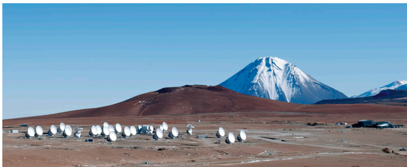
ALMA antennas and the technical building on Chajnantor.
