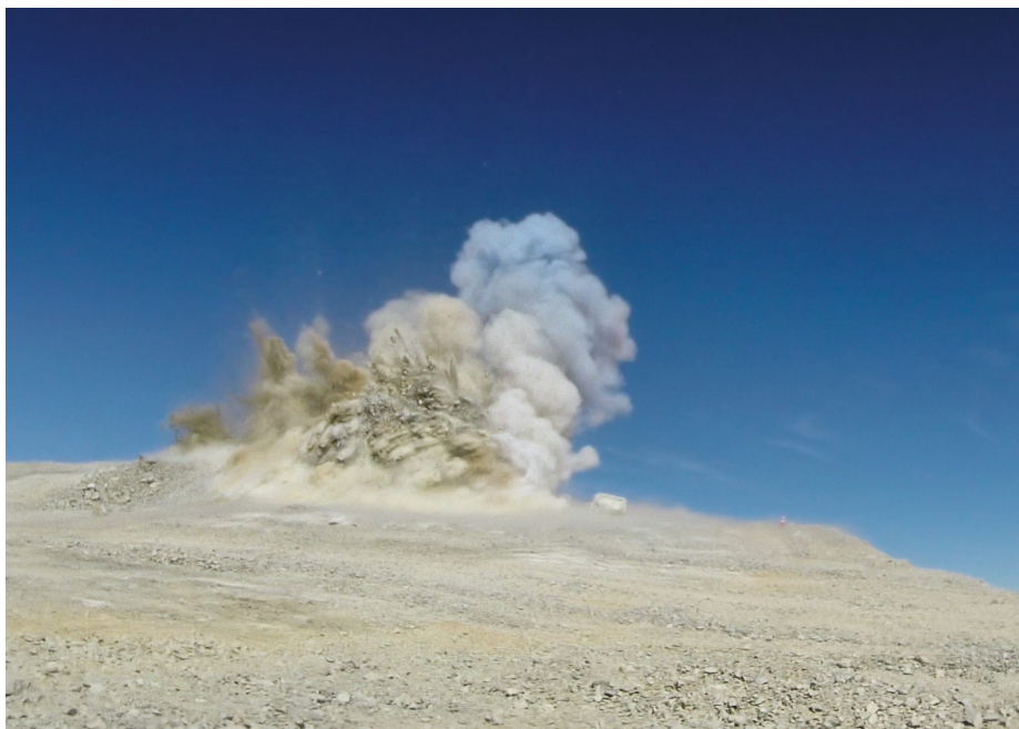
Figure 2. The moment of the explosion which loosened ~ 5000 cubic metres of the summit of Cerro Armazones, photographed from a few hundred metres distance.
