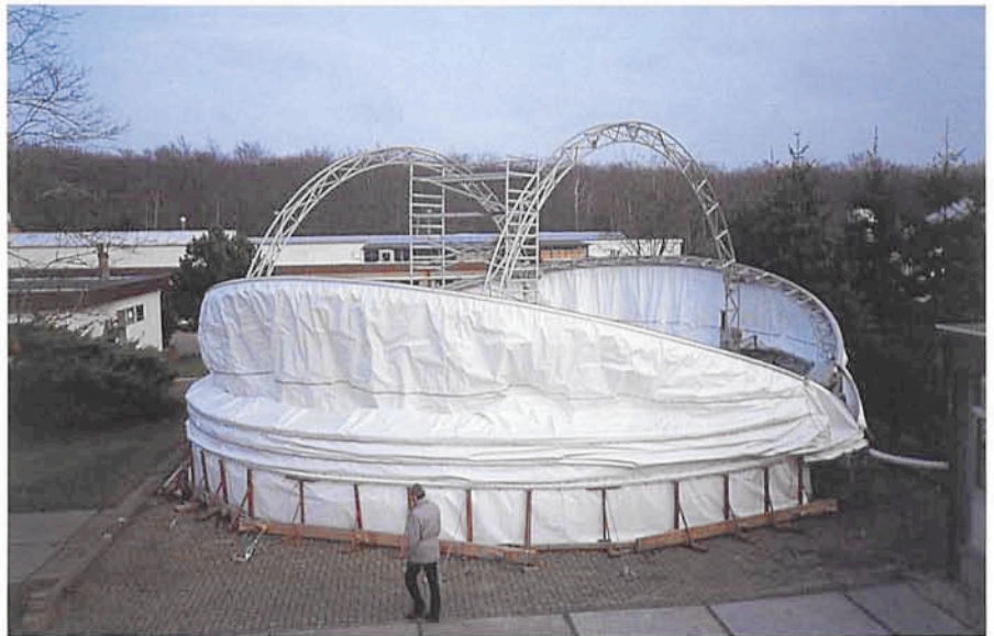
Figure 1: The 15-m dome almost open.
