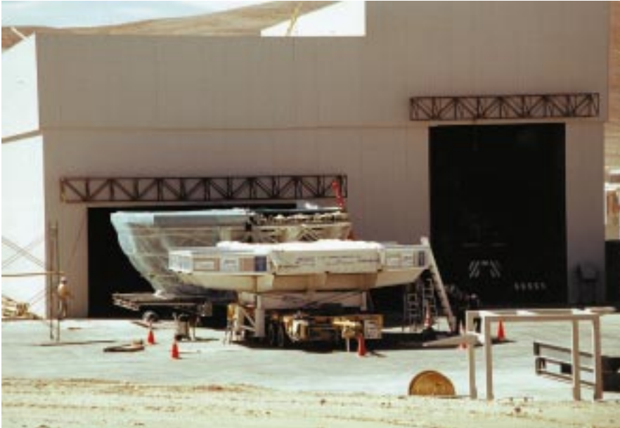
Figure 6: The M1 cell and the dummy mirror arrive in front of the Mirror Maintenance Building (MMB). Here they are being unloaded and placed next to the 10 metre wide entrance.
