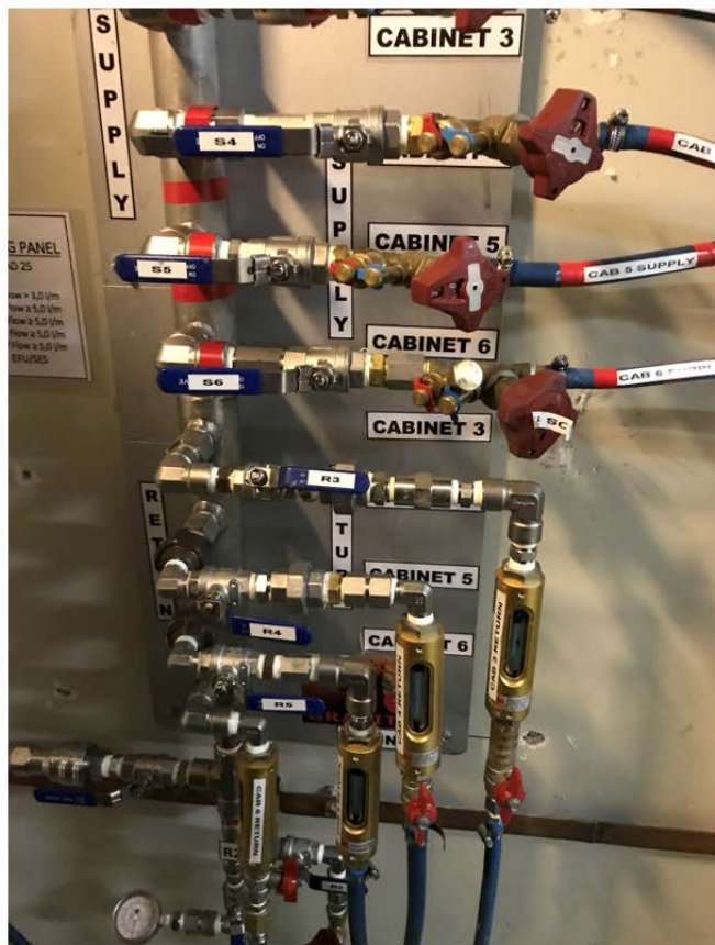
Figure 20: examples cooling fluid distribution panel in Combined Coudé Lab
