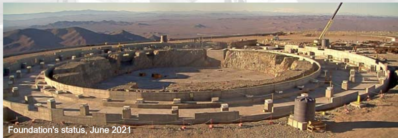
Foundation's status, June 2021
