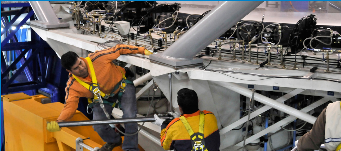
Dismounting from the telescope. 96 screws hold the mirror cell on the telescope structure.
