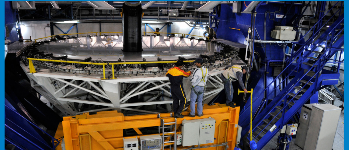
The mirror and its mirror cell (45 ton) is lowered on a special air cushion vehicle.
