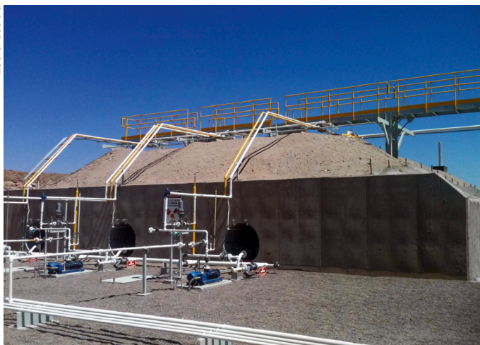
The LPG storage facility: the tanks are covered in sand for enhanced safety.
