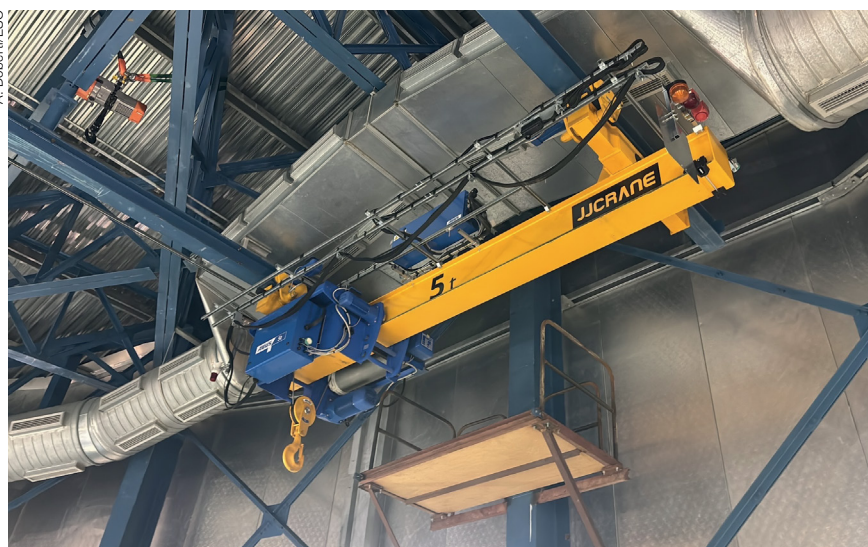
New five-tonne capacity crane installed at the VLT.
