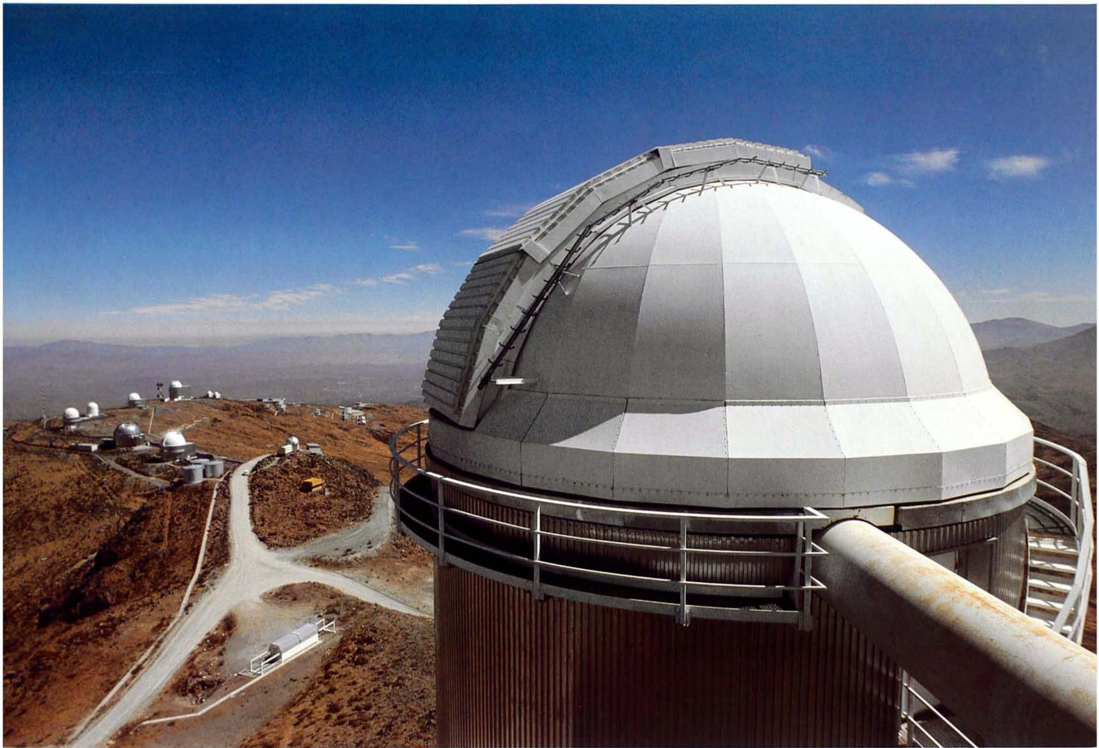
**219–220** The 1.4-m Coudé Auxiliary Telescope (CAT) is placed in a separate dome next to the 3.6-m dome, to which it is connected by an 11 m long light-tunnel. The main purpose of the  $f/32$  CAT is to feed the 3.6-m coudé instrumentation. In this way, observations can be made with the coudé spectrometer when the 3.6-m telescope itself is engaged in other work. The CAT rests in an “*alt-alt*” mounting and is driven by direct drive motors without gears.
