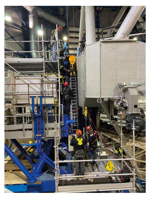
Figure 7. Implementing the upgraded cable wrap at Nasmyth B on UT2 in June 2023.
