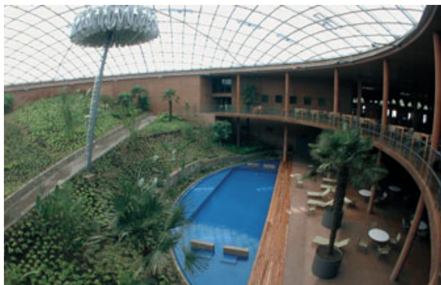
The swimming pool in the Residencia was introduced as a part of the humidification system
