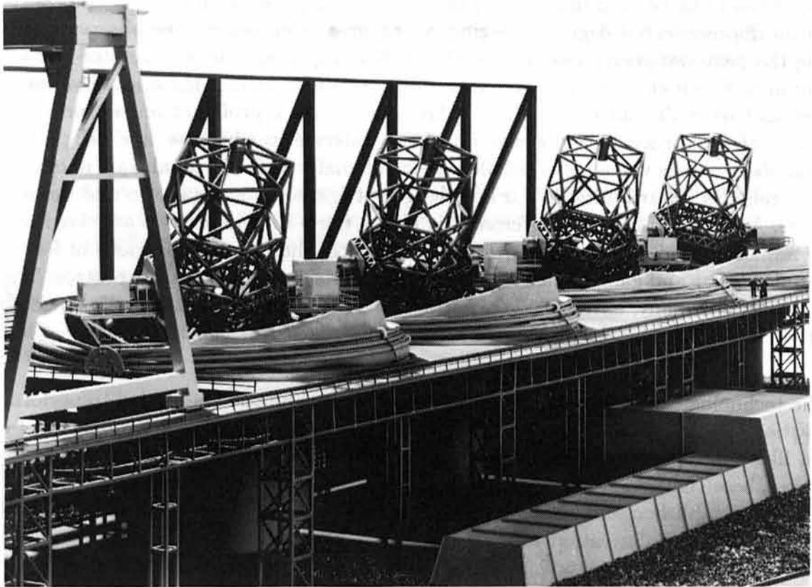
Figure 8.2: **The ESO 16 m Very Large Telescope (VLT).** The ESO VLT (here a model) consists of four connected telescopes, each with an 8 metre main mirror. They will operate in the open air and can be protected by inflatable shelters. They are served by a crane (left) that moves on a supporting platform with a length of about 120 metres. (PR 16/87; BW)
