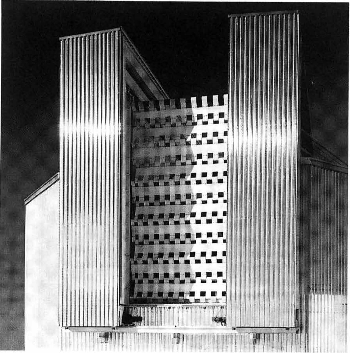
Figure 7.13: **The NTT windscreen.** During periods of high winds, the ESO New Technology Telescope is protected by a windscreen. It is elevated in front of the telescope to an appropriate height so that it does not impede the observations. In this way wind buffeting of the telescope structure is avoided and the NTT remains stable, even during wind speeds up to 70 km/h. (PR 03/90: NTT image C05).
