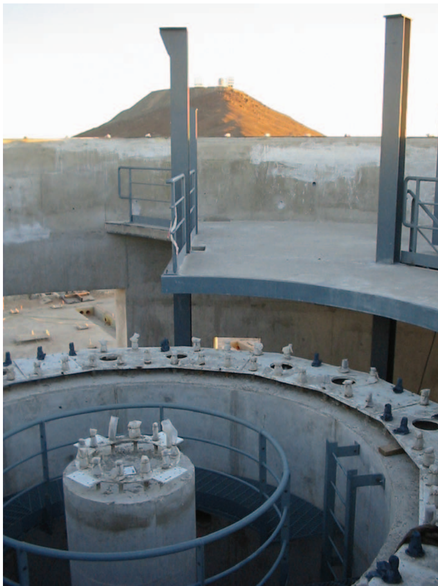
Figure 9: Telescope support base. The central column takes the azimuth encoder, the inner ring is the pier on which the telescope itself will be supported, and the enclosure will sit on the outer wall. The VLT on Cerro Paranal can be seen in the background.
