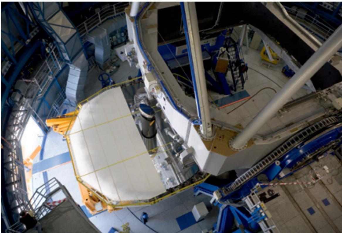
Delicate manoeuvres in the daylight. The 8.2 m primary mirror of VLT Antu (UT1) being removed prior to aluminization in December 2005. The white screen covering half of the mirror prevents direct sunlight from the open dome door falling onto the mirror during removal from the telescope.
