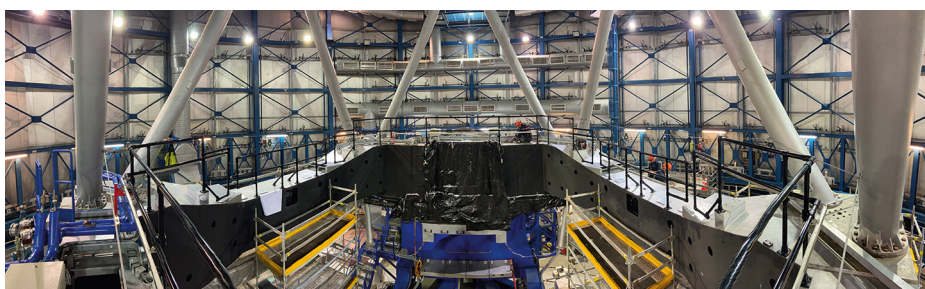
Figure 4. UT2 centrepiece at the end of the intervention in April 2023.
