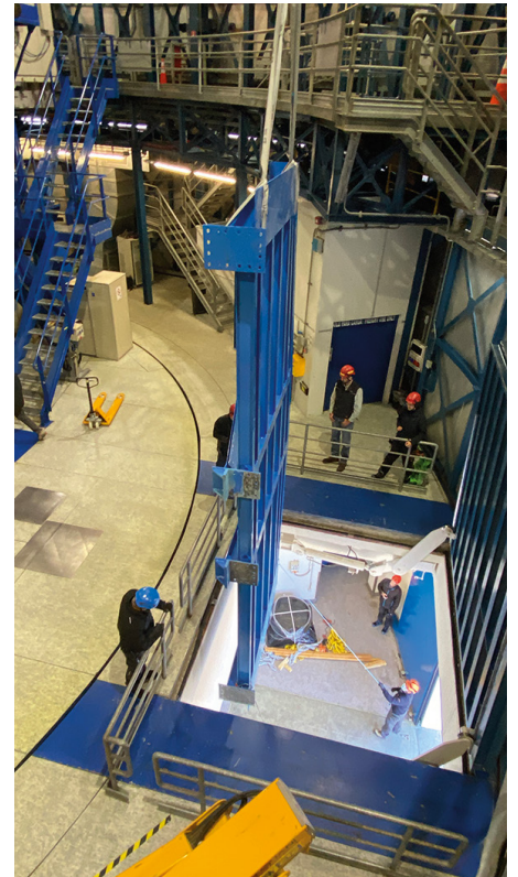
Figure 8. Transfer of the largest part of the sub-Nasmyth platform B on UT2 in June 2023.
