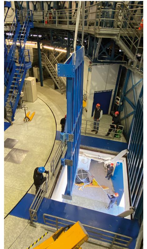
Figure 8. Transfer of the largest part of the sub-Nasmyth platform B on UT2 in June 2023.
