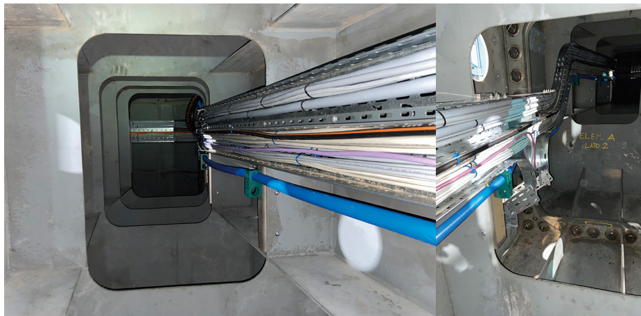
Figure 5. Inside the centrepiece of UT1 in August 2023.
