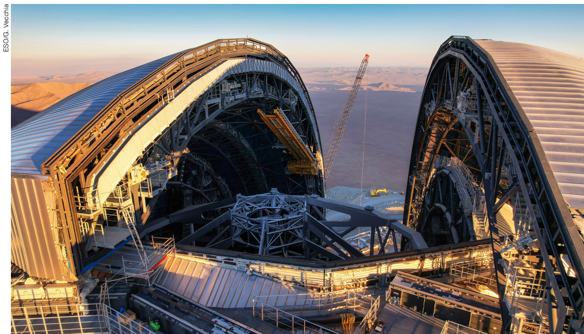
This drone image, taken in April 2026, shows a stunning view above the dome of ESO's Extremely Large Telescope (ELT), under construction atop Cerro Armazones, a mountain in Chile's Atacama Desert. The sliding doors are partially open, showing the top of the telescope's main structure inside. The catwalks running along the edges of the sliding doors convey the sheer size of the 80-m high dome.
