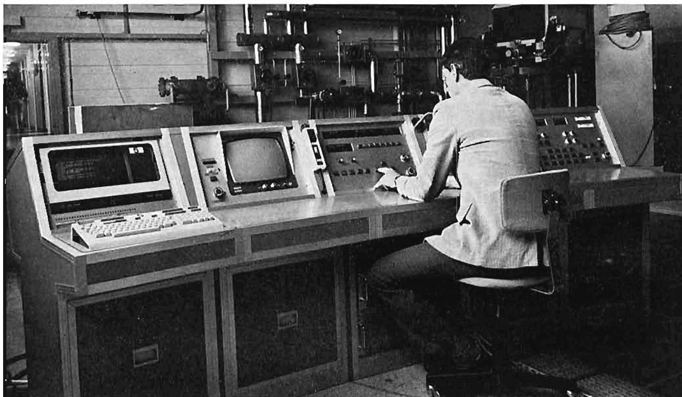
Main desk of the ESO 3.6 m telescope control system in the ESO assembly hall before departure to La Silla.
