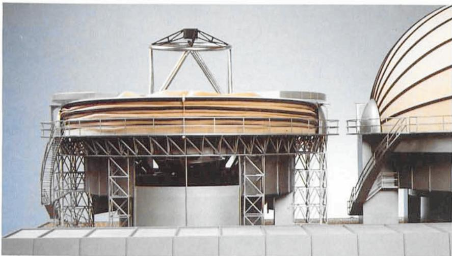
Figure 4: The enclosure in open configuration.
