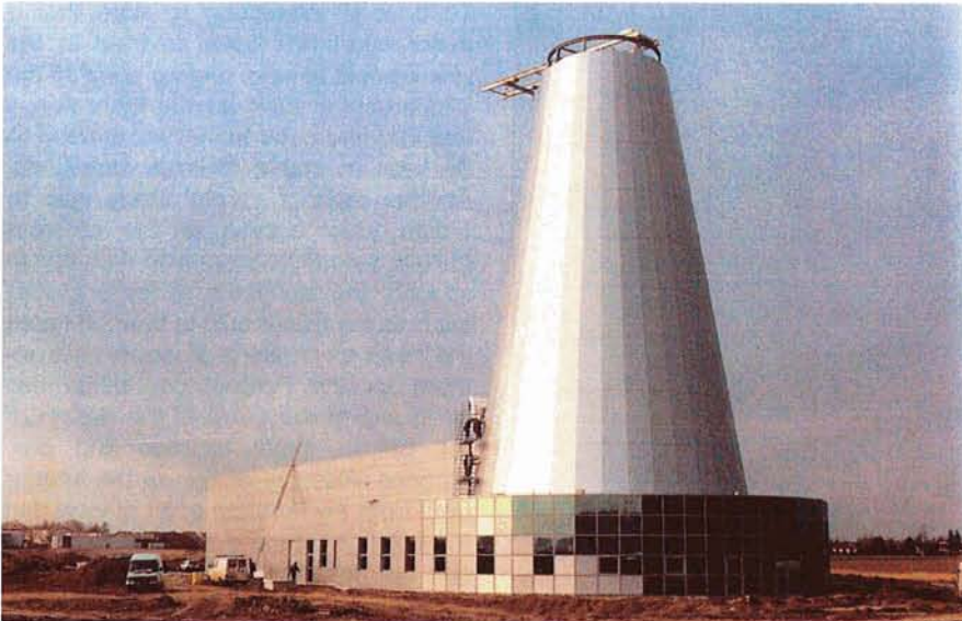
Figure 1: General view of the shop with the 32-m tower. In the foreground are the meeting room and the offices. On this picture, the sunshield is under achievement and the tower has not been topped with the 4-m dome.
