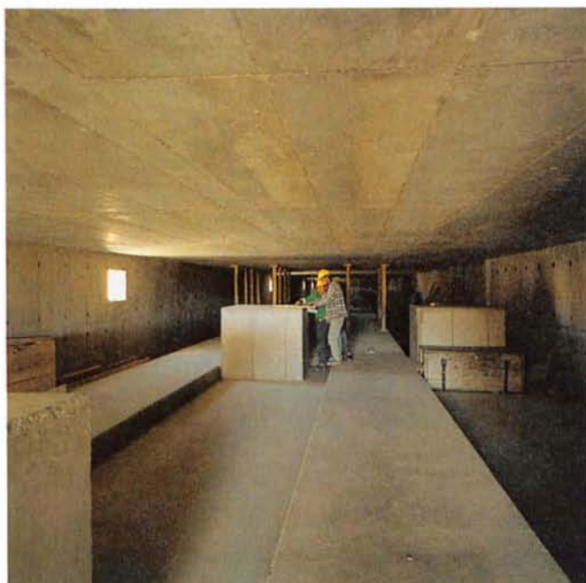
Figure 4: The completed section of the delay line tunnel.
