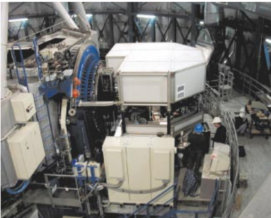
Figure 1: This aerial view of the Nasmyth platform of Kueyen at the end of the integration shows UVES with the top of its enclosure partially lifted to have access to the table where the various components are mounted. The bar connecting the enclosure to the telescope fork is for safety in case of earthquake.
